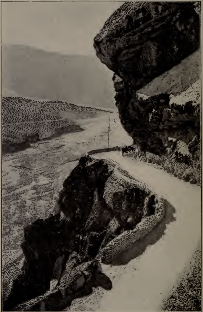
Section of the road in Darial Pass
